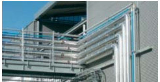
Outdoor installation Transair Ø 168
